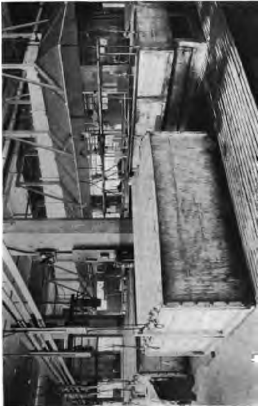
Fig. 1. Nickel Plating Dept., Eastman Kodak Company. Note arrangement of exhaust system for carrying off acid fumes and steam, also method of covering tanks.
